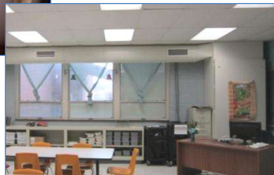
New energy recovery heat pump
