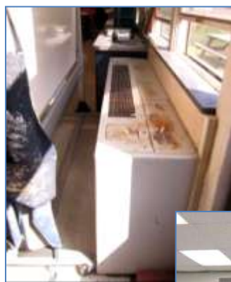
1950's era steam unit ventilator/heating unit.
